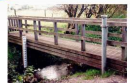
water level measurement with pressure sensor
